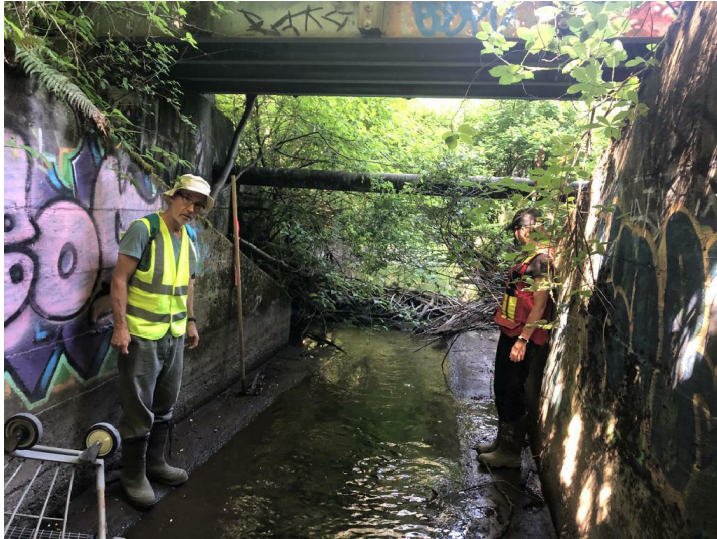
1.) Placemark 3- Reach 2 Culvert under Highway 1.
