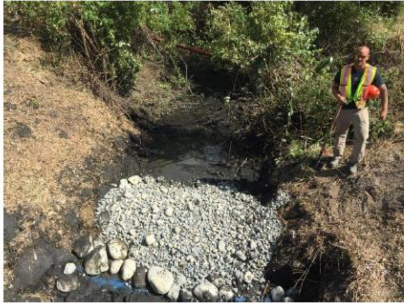
Swan Creek installing gravel/crests at low flow
