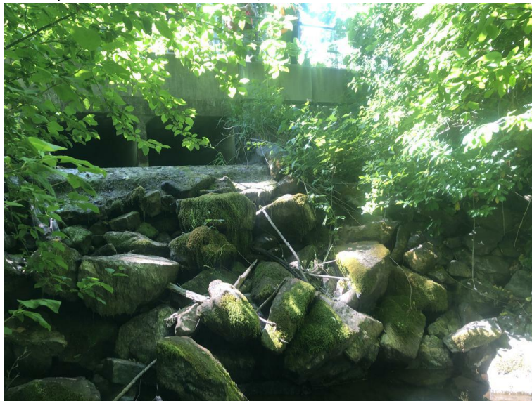
3.) Placemark 32-Reach 5 end at Somenos rd. - Fish passage barrier.
