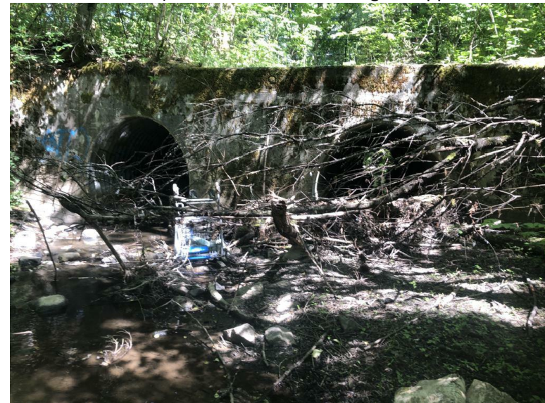
4.) Placemark 32- R3 end; culverts at the confluence with Raphael Creek.
