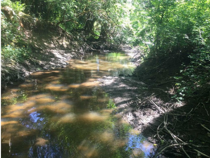
R3 –Pool 6 full of fines and heavily eroded, unstable banks
