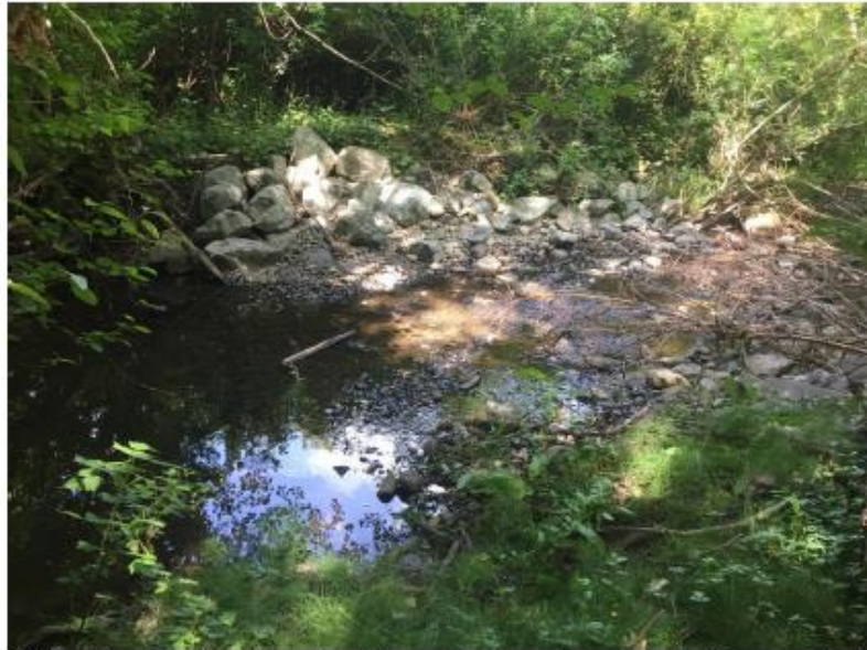
Averill Creek – looking d/s note wide anchor crest apron to hold gravel in place.
