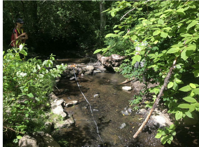
R2 –Failing riffle crest from previous restoration.
