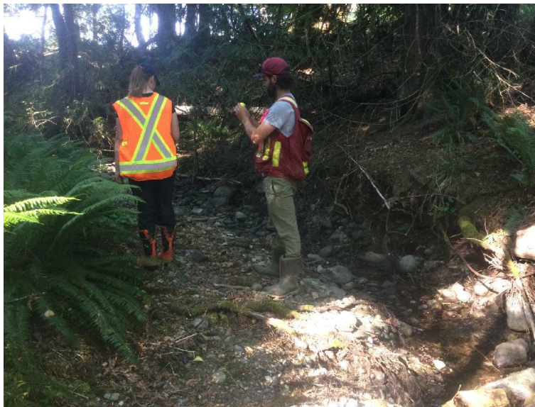
3.) Upper reach, bank erosion through golf course.
