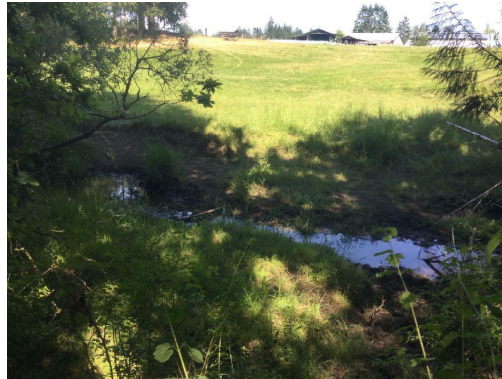
4.) Reach 4, eroded banks from livestock access.
