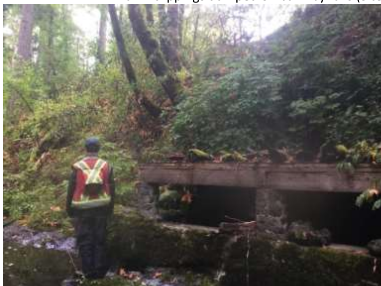
R4 - Site 46, decommissioned water inlet, no concerns.
