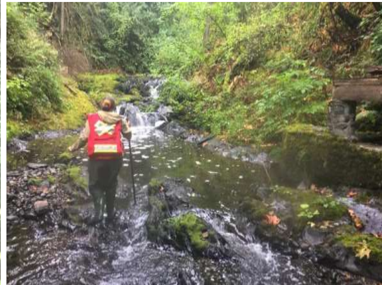
2.) R4 below falls 2 is old water inlet structure
