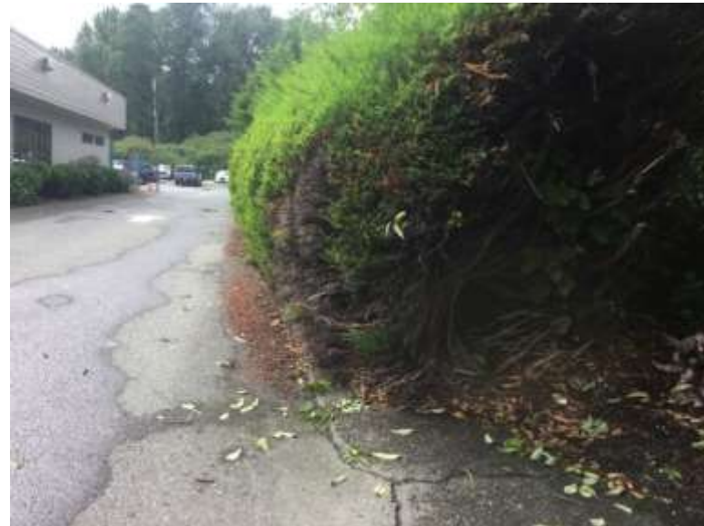
2.) R2 Site 118 –RCMP property is channelized, close to pavement.
