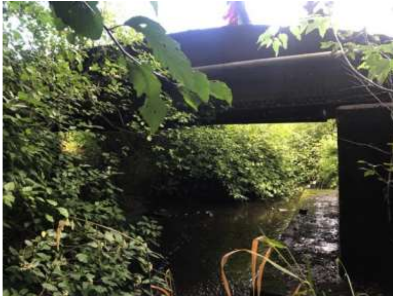
1.) R2 Site 117, E&N Bridge
