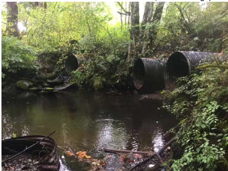
R6. Hung CV Trail culverts near Cleve Road (Site 94)
