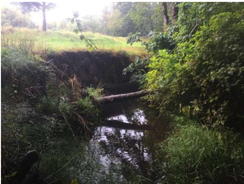
R6 – Farm Bank Erosion from blowdown/undercutting (Site 88)
