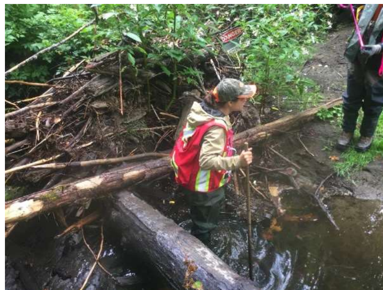
2.) R3 Site 33 log and debris jam
