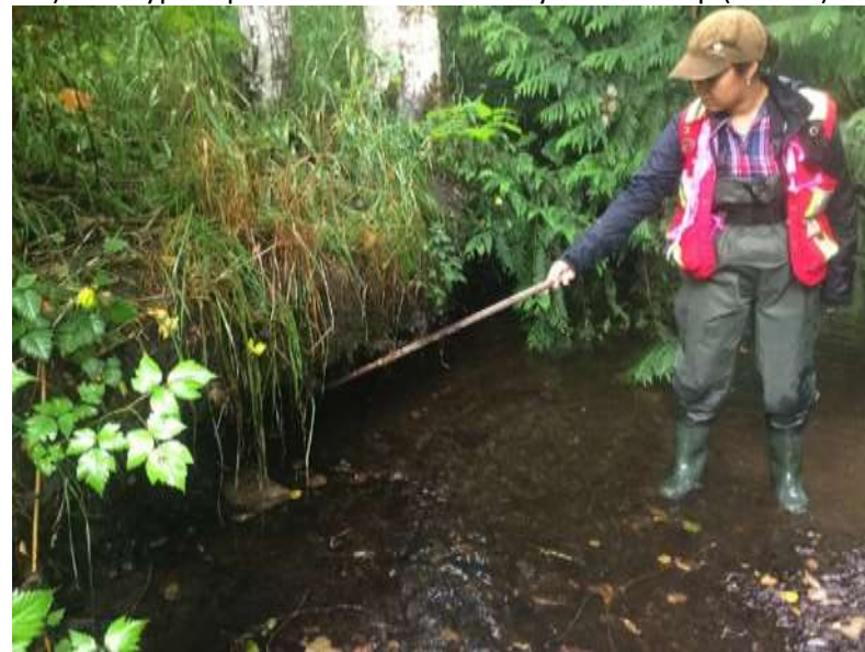
4.) R6- Undercut bank offers cover but lacks root structure. (Site 89)
