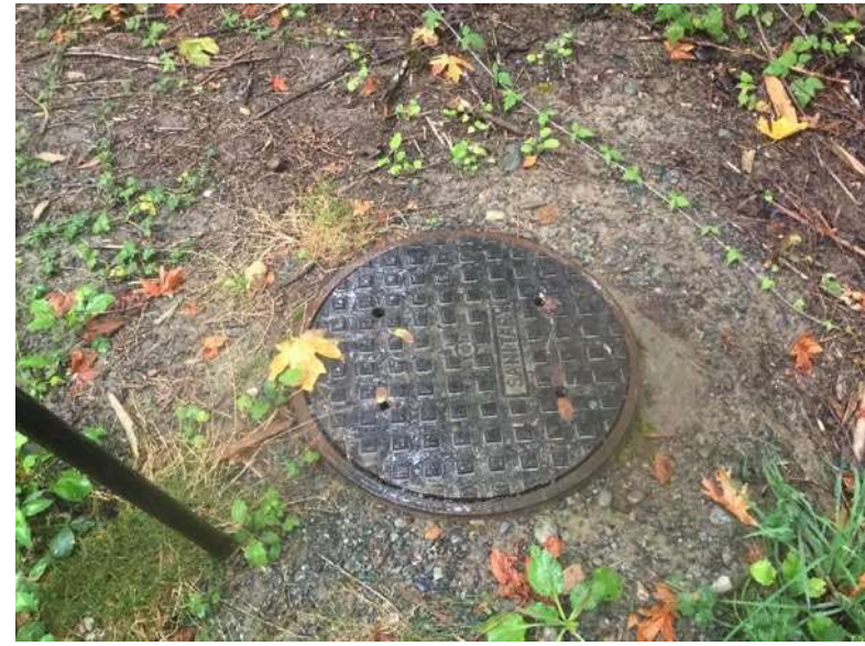
R5 –Sewer line runs parallel Creek. (Site 69 near Keystone)
