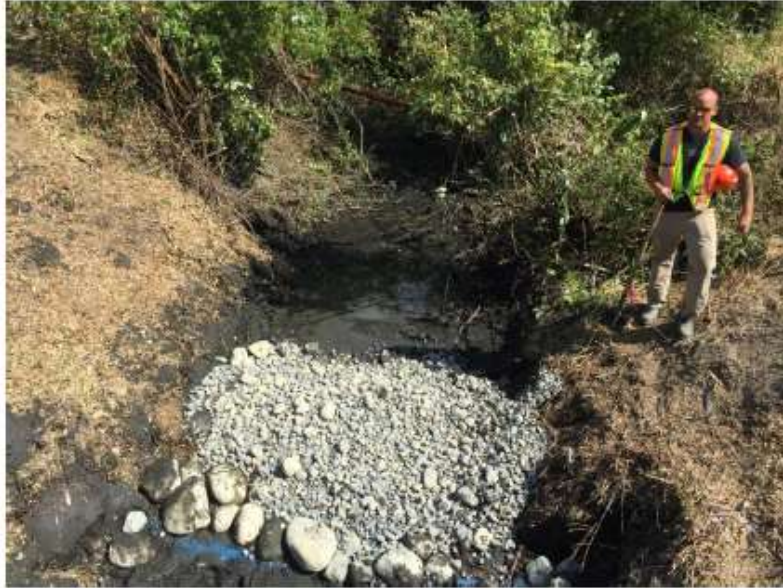
Swan Creek installing gravel/crests at low flow
