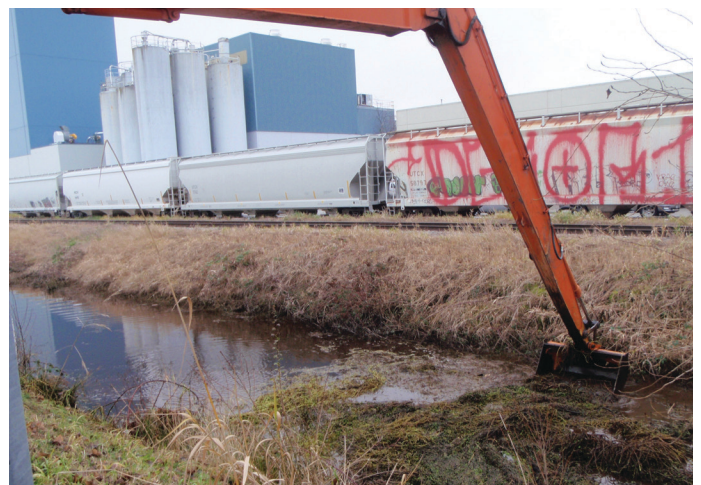
Excavation of parrot's feather in ditches in Richmond
