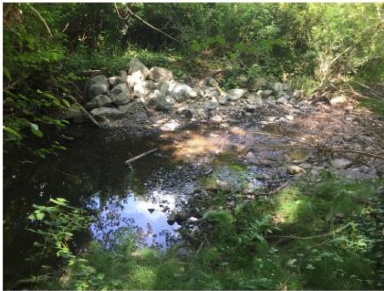
Averill Creek – looking d/s note wide anchor crest apron to hold gravel in place.
