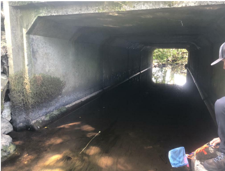
R2 – Box culvert at Richards Trail
