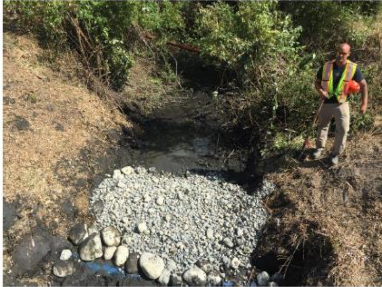
Swan Creek installing gravel/crests at low flow
