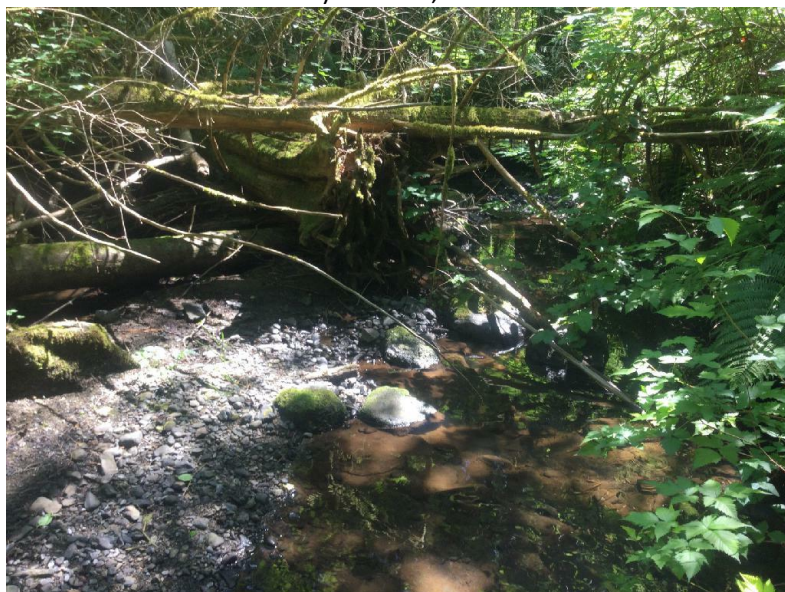
3.) Reach 3, Pool 4 Debris Jam
