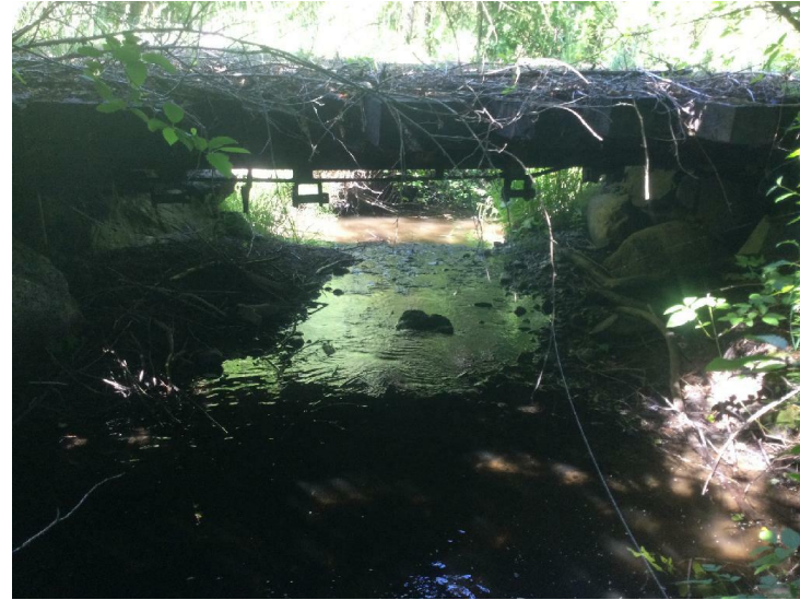
2.) Reach 2, Riffle 3- Riffle under old farm bridge.
