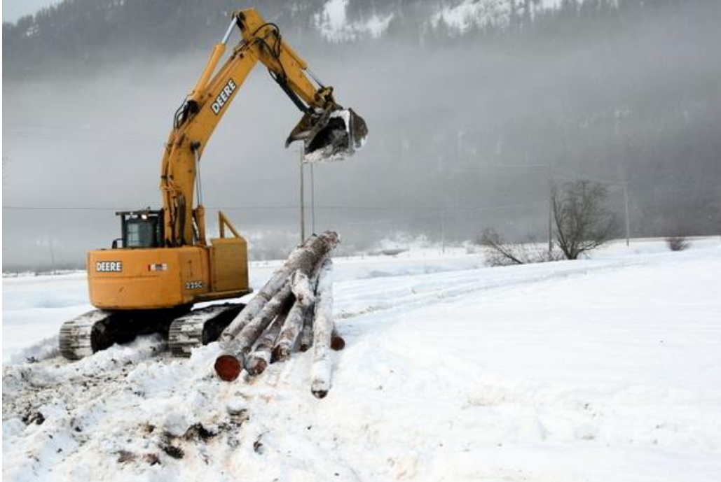
The excavator can move logs to the worksites
