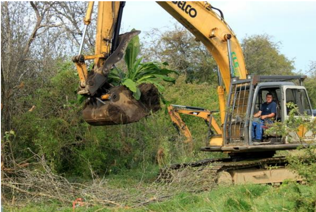
Desirable native plants such as skunk cabbage would be removed, saved, and replanted in the restored wetlands. This skunk cabbage was growing along the edge of a drainage ditch.
